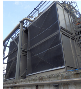
Air Inlet Screens Keep the tower interior free of leaves and debris.
