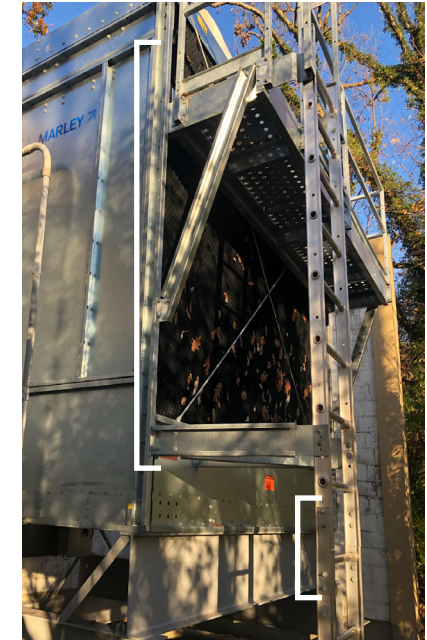
Louver Face Platform (Platform can be located as pictured to clean HW Basins or at CW Basin level to ease cleaning of fill or CW Basin.)
